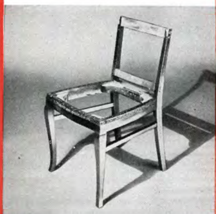
Cut down the back to 32 in., screw cross pieces across back, strengthen joints with angle irons, cut an inch from legs
